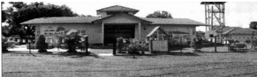
Figure 1.2: Front view of new preschool building (annex building) with two classrooms
