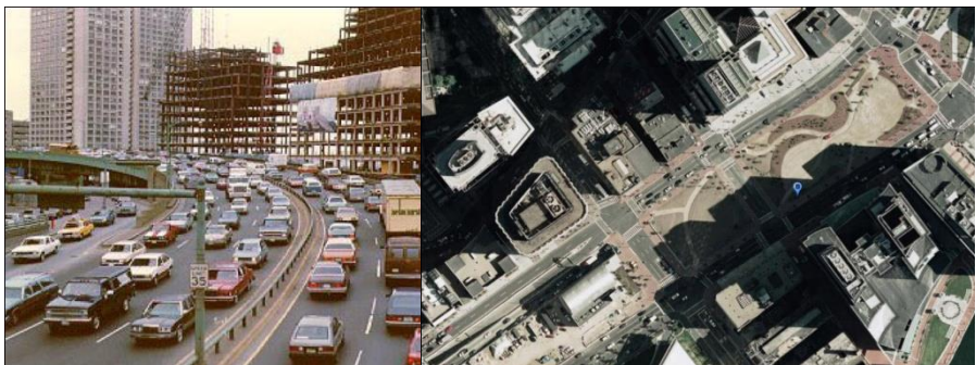
Fig. 3. Boston John Fitzgerald Expressway - Central Artery, before & after the project (BECT/AREP, 2009)
