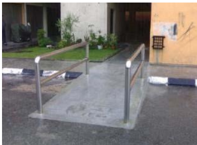
Figure 3: Ramp into a Building at a Low Cost Housing
