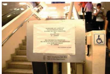
Figure 9: A Notice Instruction on a Typed Small Piece of Paper on How to Use the Platform Lift, Clearly Lacking in Contrast and Font Size to Read for PWD (Source: Authors, 2011)
