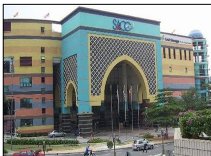
Figure 4: Shah Alam Commercial Complex, Selangor Malaysia
