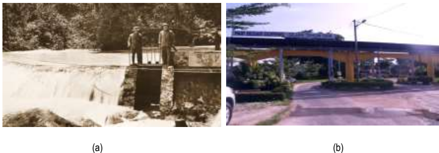
Fig. 2. (a) Ulu Geroh Dam, Gopeng; (b) Gopeng giant pipes
