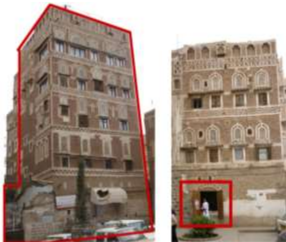
Fig 4. Indication Of The Space Of Adaptation On The Tower House, Left Side Fully Adaptation, Right Partially
