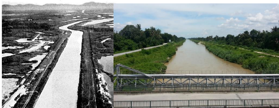
Figure 2: The canalization of Kinta River involving 61km length, from Ipoh to Kuala Chenderiang. Source: Old photo reproduced from (Khoo & Lubis, 2005, p. 325); new photo was photograph by author in 2018.
