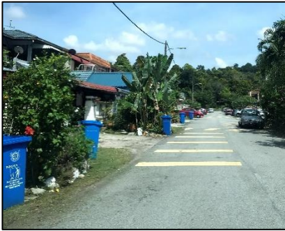
Figure 12: State of waste landed houses, Seksyen 6 (Source: Researcher, 2020)
