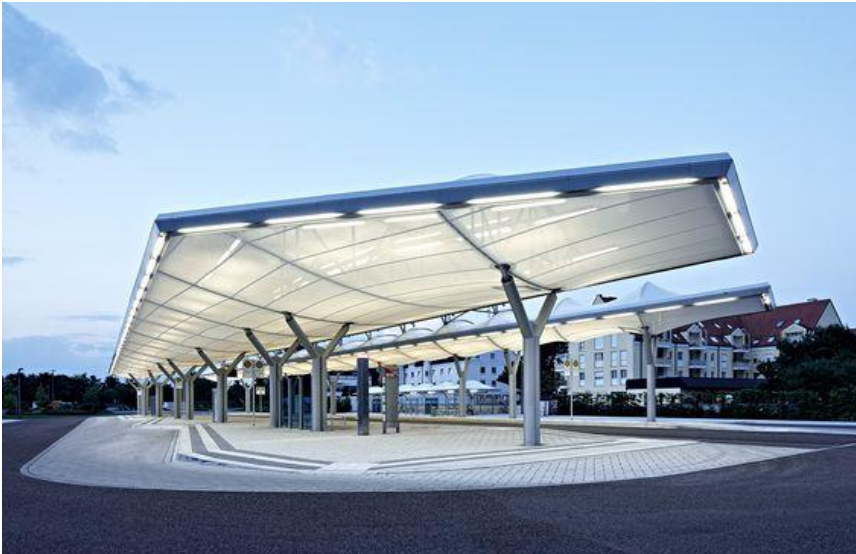
Figure 1: PVC-coated polyester membrane roof (Bus Station Konigsbrunn) (Source: www.pinterest.com )
