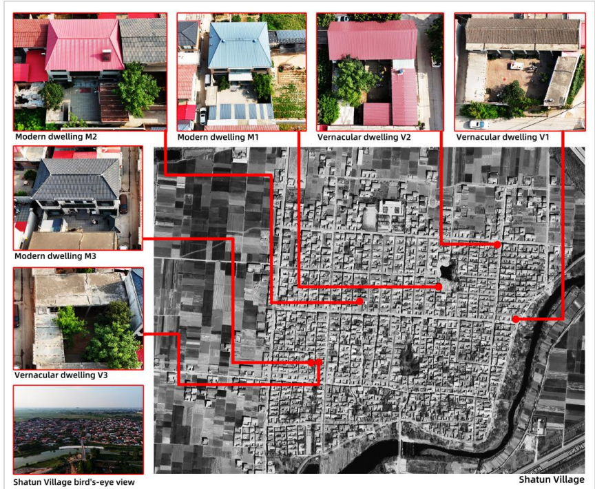
Figure 2: Study area location and the condition of houses in the surveyed village
